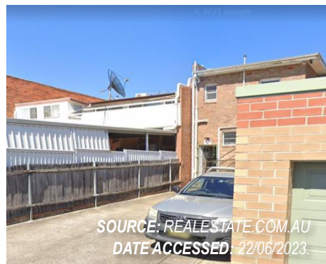
FIGURE 4: VIEW OF REAR CAR PARK
