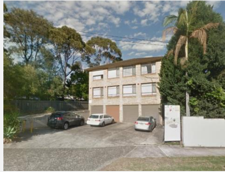
FIGURE 8: VIEW OF 297-299 A3, ROSELANDS NSW 2196 ADJACENT TO THE NORTH
