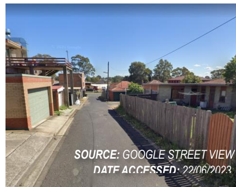
FIGURE 5: REAR VIEW OF MOOREFIELDS LN LOOKING EAST
